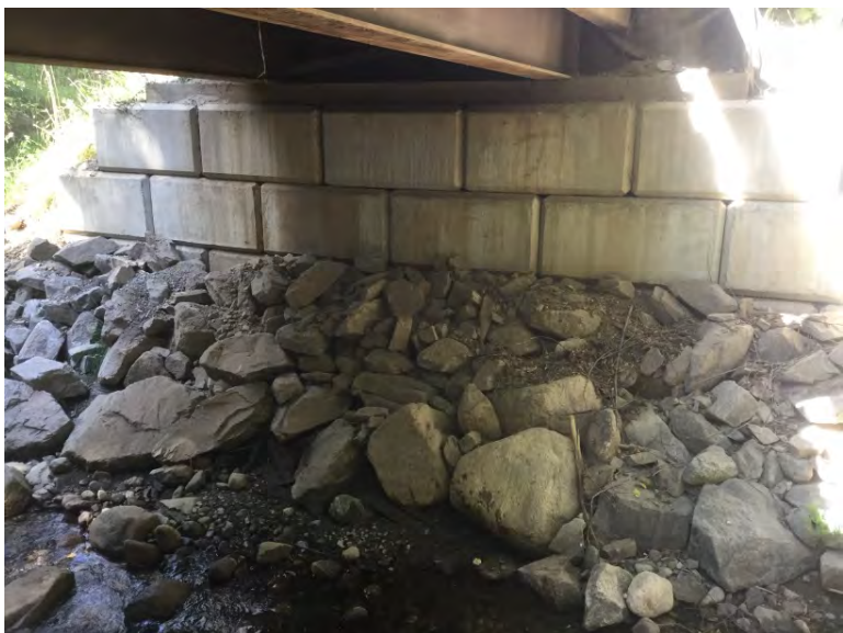
Right Bank Abutment when facing downstream
