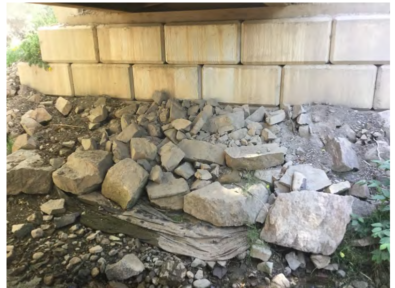
Left Bank Abutment when facing downstream
